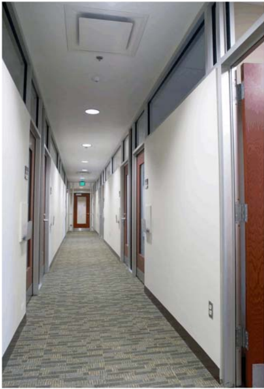
.DAB0564 Krannert school of management third floor renovation of Krannert undergraduate facilities.
